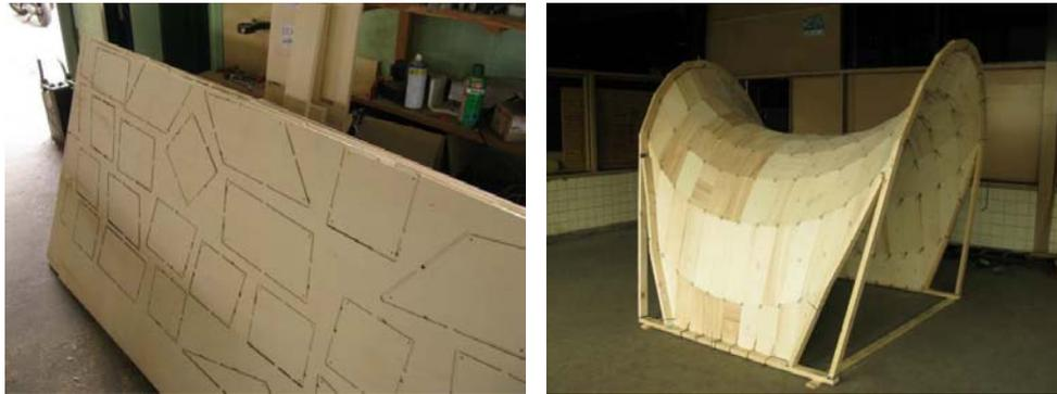
**Figure 2. A form active membrane structure, built with solid components. Similar to clothing, desired developable shapes can be cut out of the building material and assembled together by joints and seams to create a whole (Vrouwe et al. 2011).**
