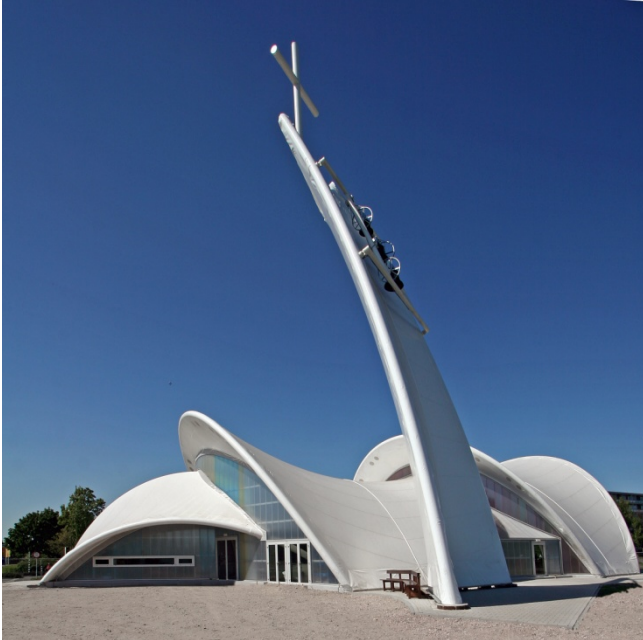
Figure 2. Petrus and Paulus Church Maassluis, Architect: Haskoning Architects, Membrane engineering: Tentech B.V. An example of membrane design and engineering by the researcher.
