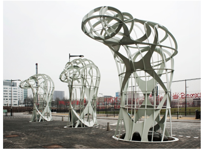
Figure 6. Pergola, Artist: Arjan Karssen, Structural Design and Engineering: Mark Feijen, Ivo Vrouwe. An example of Phase 2; Volume patterning reframed into a section-active system by the use of steel.
