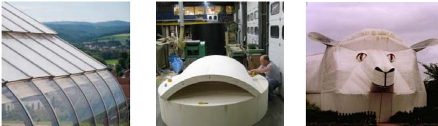
Figure 1a,b and c: “cold” bent Plexiglas in *Bio Solar Haus* in Germany; “cold” bent laminated wooden panels for stage setting of Barbara van Loon; “cold” bent corrugated steel panels (partly) in sheep shaped artwork in New Zealand
